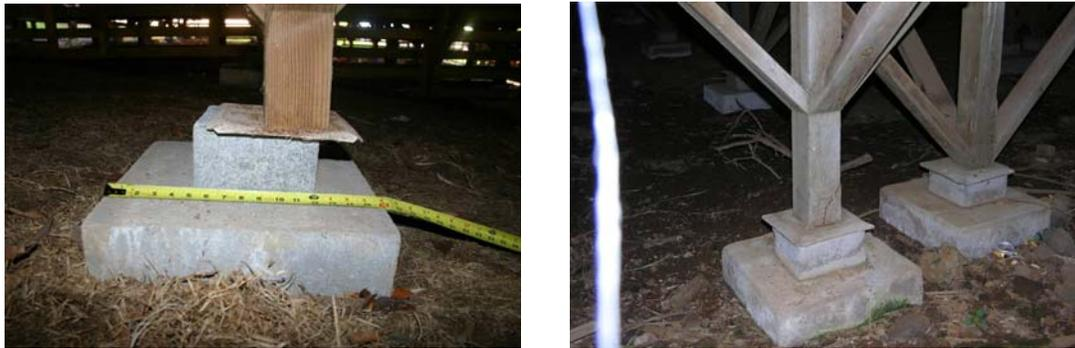
Figure 5. Shifting (left image) and cracking (right image) of foundation elements.
