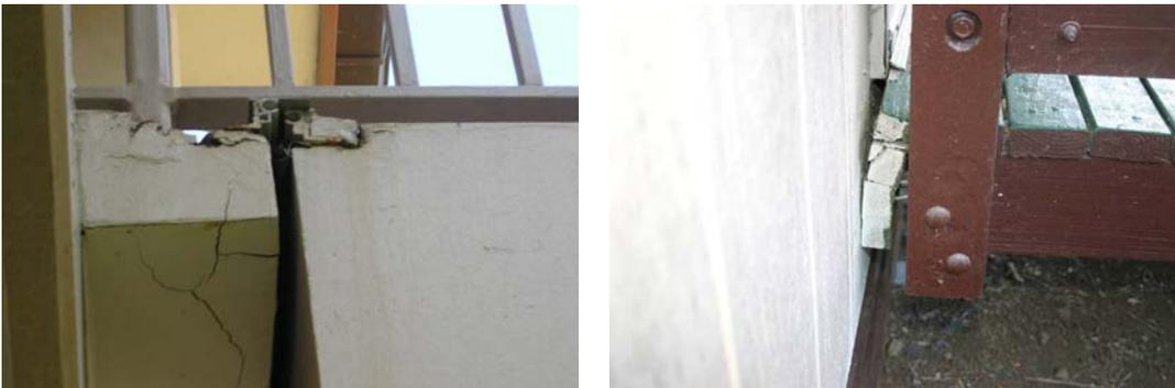
Figure 8. Damage due to differential movement of elements.
