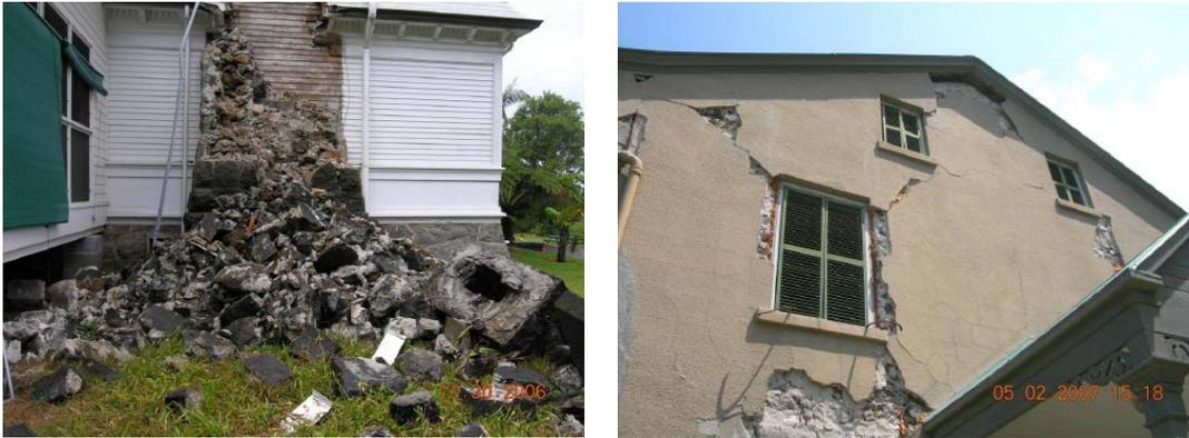
Figure 7. Damage to cement rubble masonry elements.
