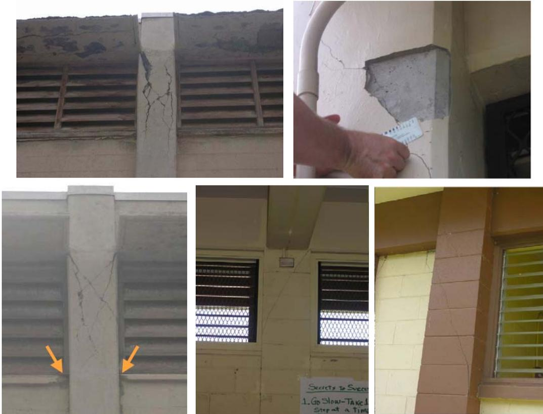
Figure 3. Classical shear cracking of short columns.
