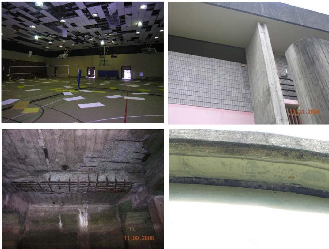
Figure 10. (Top left) ceiling tiles and suspension system; (top right) infill wall damage; (bottom left) spalling of concrete cover over corroded rebar; (bottom right) lateral displacement of concrete water tank roof.
