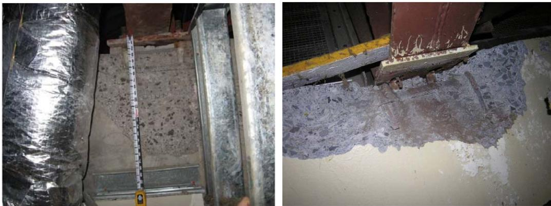
Figure 4. Cracking/spalling at bearing area of beam/truss. Note corrosion of embedded reinforcement.
