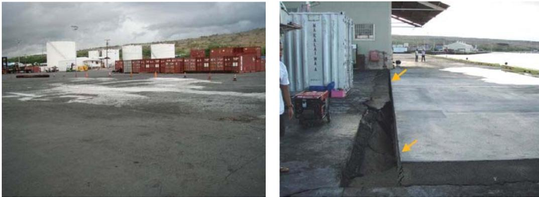
Figure 9. Evidence of sand ejecta (left), structural damage due to shifting of building foundation (right).
