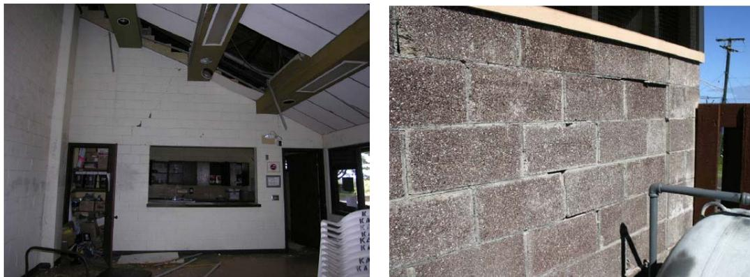
Figure 6. Examples of cracking and shifting of CMU block walls.
