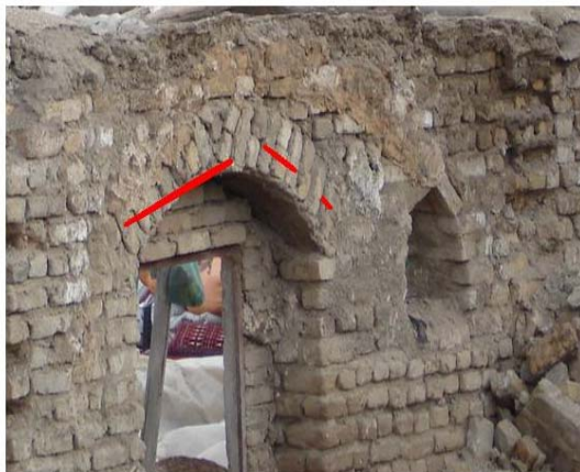
Figure .6: Brick lintel
