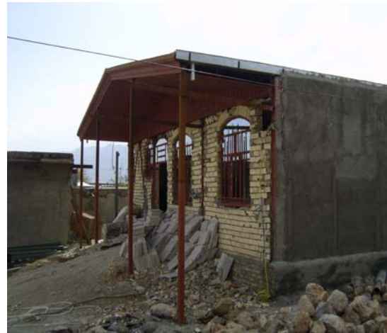
Figure 8: Reconstruction/Renovation design with a sloping roof & terrace
