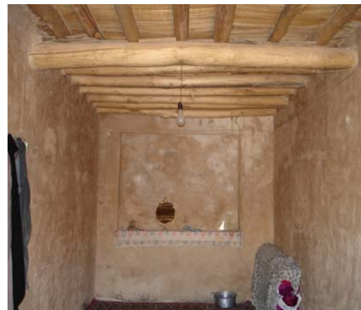
Figure 4: Roofs with wooden beam covering: These are made of straight white wood and are placed in an orderly manner at a measured distance from one another. In this kind, the primary (main) beams are vast in number, whilst the secondary ones are placed cross wise upon them
