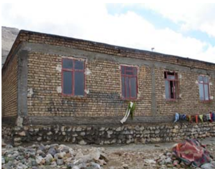
Figure .1 Stone foundations laid under brick walls with chenage are constructed with new material before and after an earthquake
