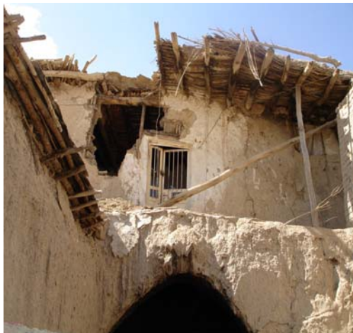
Figure 3 :Sis Roof: This kind of sis roof in the shape of an arch is made of clay and mud. The reason for selection of this kind is due to the suitable nature of the arch in resisting and shifting of pressure. Since these roofs are usually made on the lower floor, the elevation is increased in order to have a flat surfaced ground floor
