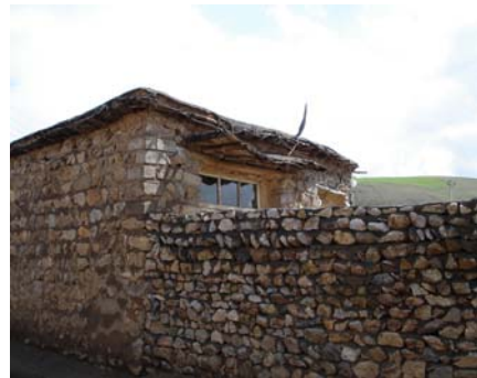
Figure .2 Stone walls are built of stone, sand and cement. These walls, due to climatic conditions should have hooks (chenage), in addition the walls' vertical joints (mortar joints,) should be filled in completely
