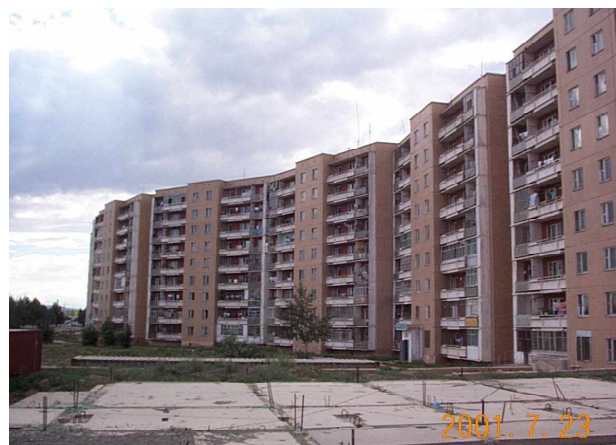
Fig.8 A typical pre-cast panel buildings in the suburb of Ulaanbaatar as residential apartments
