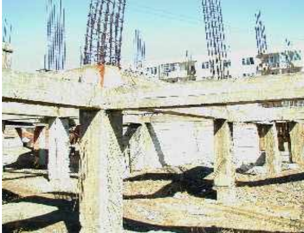
Fig.9 A cast-in-place reinforced concrete building under construction.
