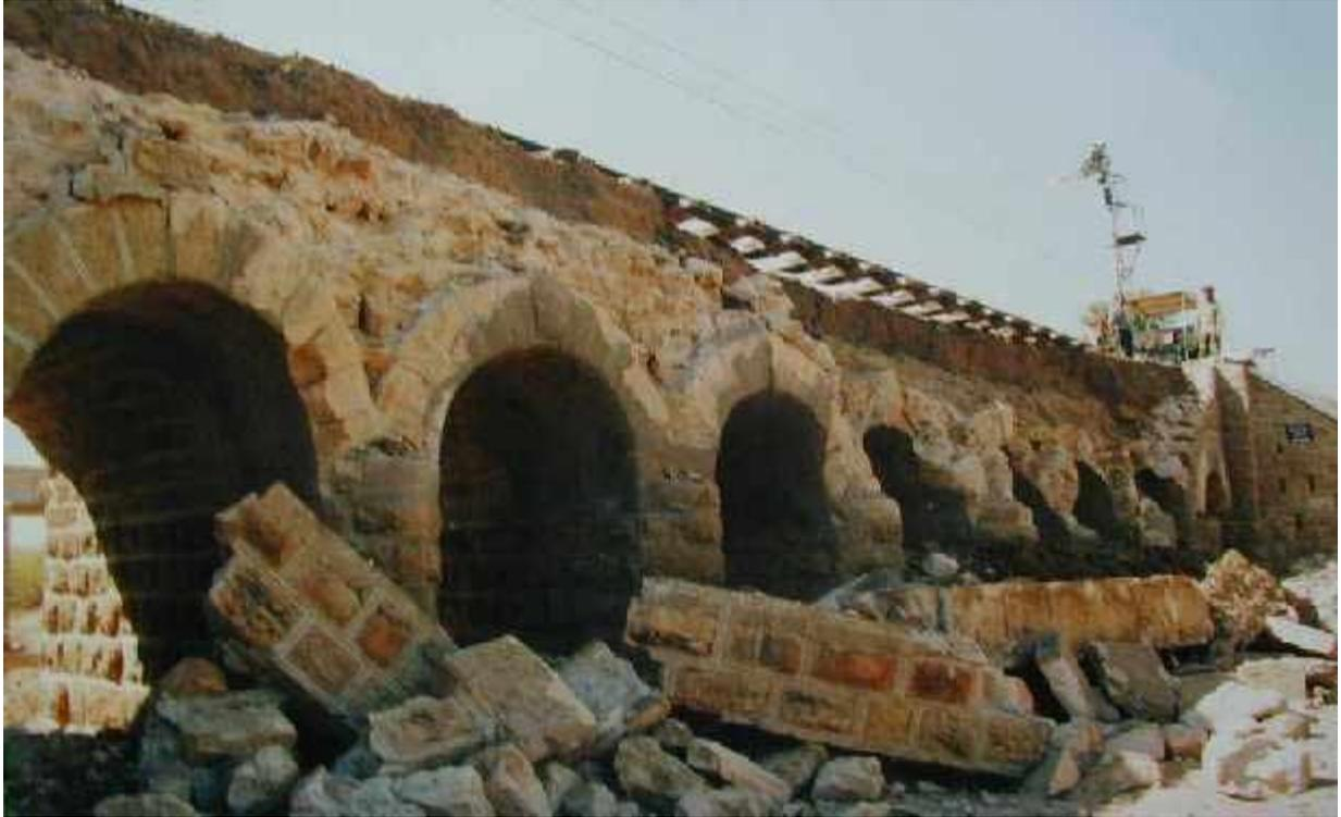
**Figure 4. Failed spandrel walls of masonry arch bridge. *Western Railways (India) photo***
