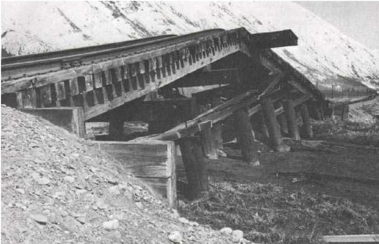
**Figure 3. Vertical buckling of trestle caused by lateral spreading.**
