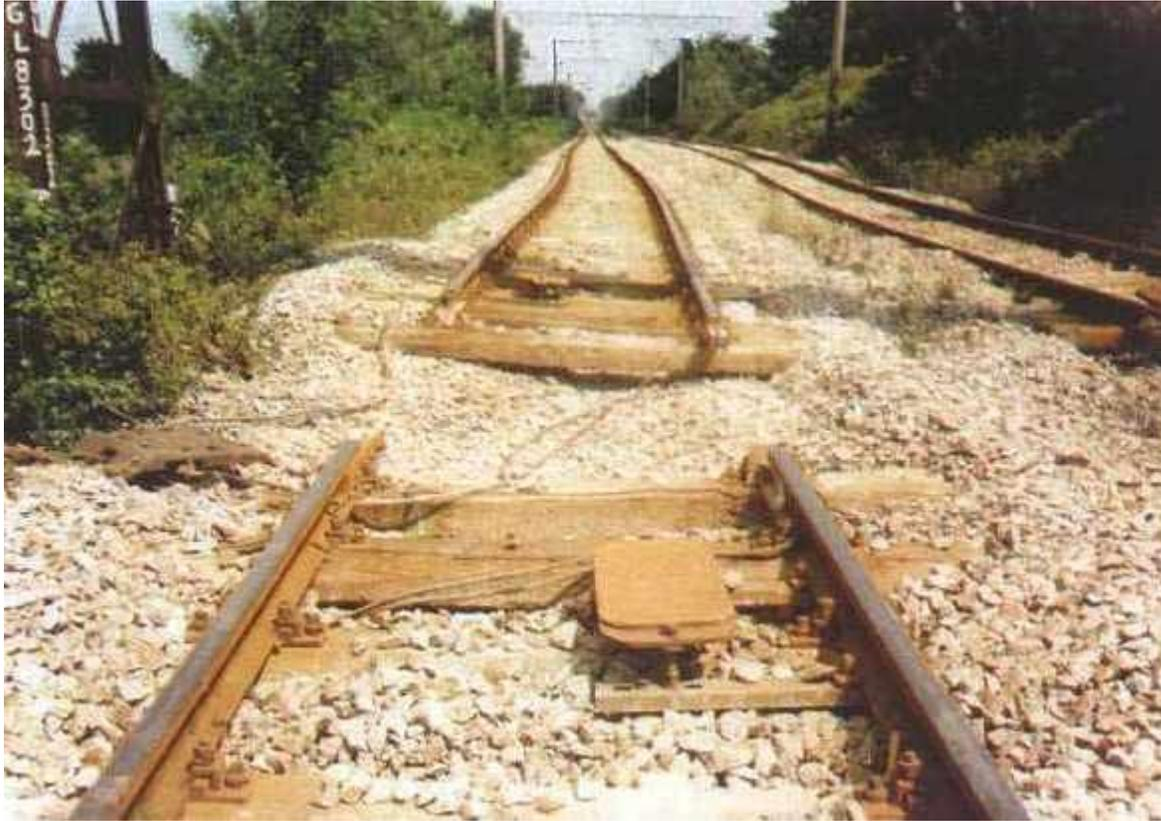
**Figure 5. Insulated joints pulled apart by ground motion. *Turkish State Railways photo***
