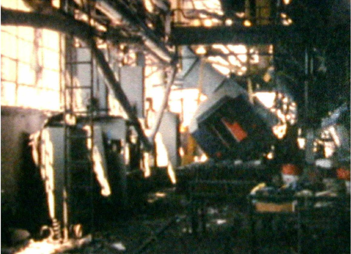
**Figure 7. Car partially overturned by failed structure in Adapazari shop.**
