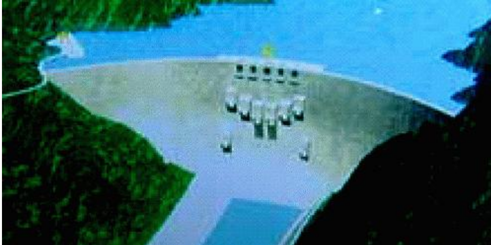
Fig.3 General view of the Xiaowan arch dam (in design)
