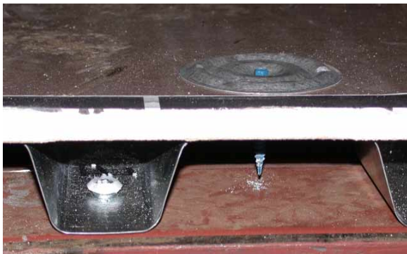
Figure 8: Gypsum board-to-deck fastener layout.
