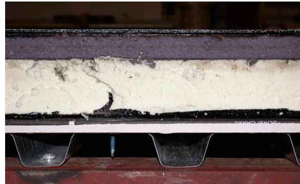
Figure 11: Cross Section View of Roofing Completed Diaphragm Test Specimen.
