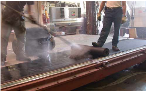
Figure 10: Installation of Non-Structural Components.
