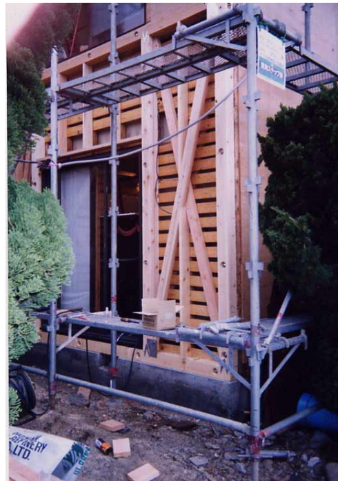
Photo 4 Construction For Strengthening
