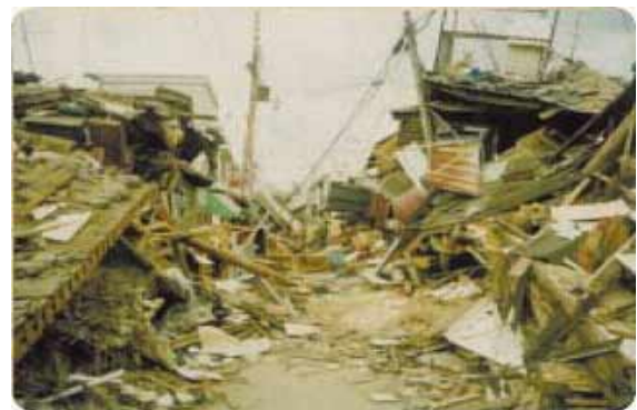
Photo 2 Collapsed houses in Hanshin-Awaji Earthquake
