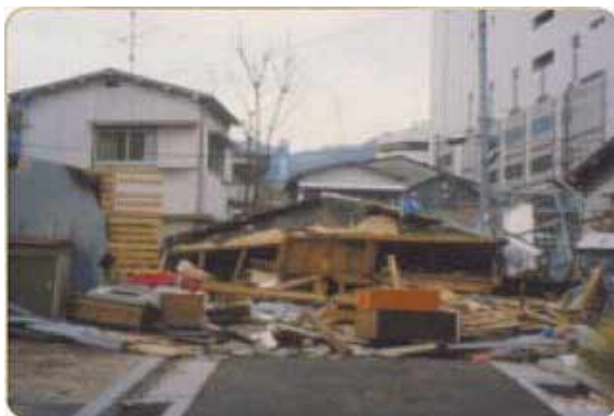
Photo 1 Collapsed houses in Hanshin-Awaji Earthquake
