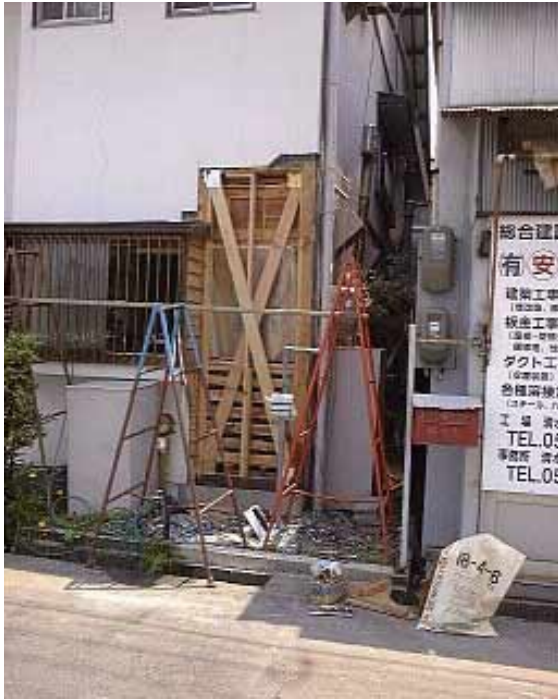
Photo 3 Construction For Strengthening
