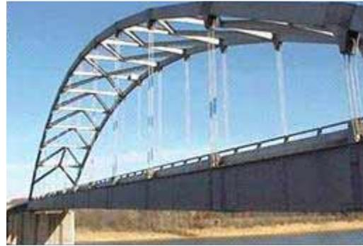
( b ) Side view of a tied-arch main span
