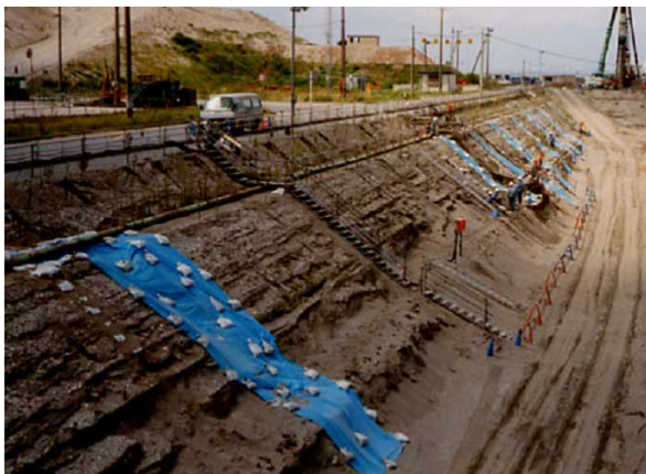
Fig.1 Excavation slope in reclaimed ground showing lamination of sublayers
