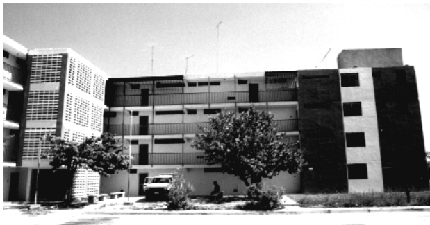
Figure 11: View of the repaired south facade of the building "Los Bloques" (photo taken in 1999)
