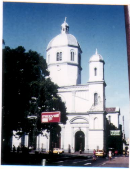
Photo 1. Facade of La Pobreza Cathedral.
