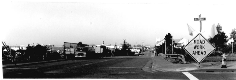
c) View of deck of 11th Street Overpass
