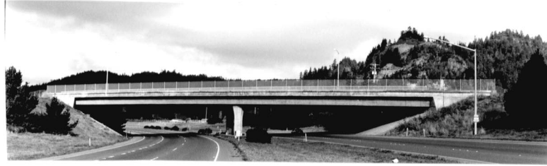
a) Painter Street Overpass
