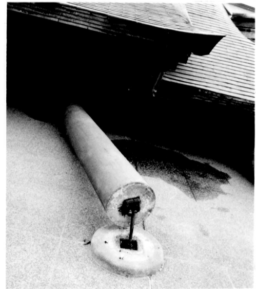
Photo.2 Bottom part of the column
