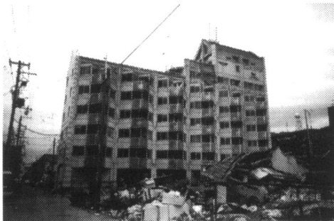
Photo 3.a A panoramic view of an eight-story RC housing building showing the joint damage in different locations Photo 3.b. Close-up view of the damaged joint condition at the reentrant corner
