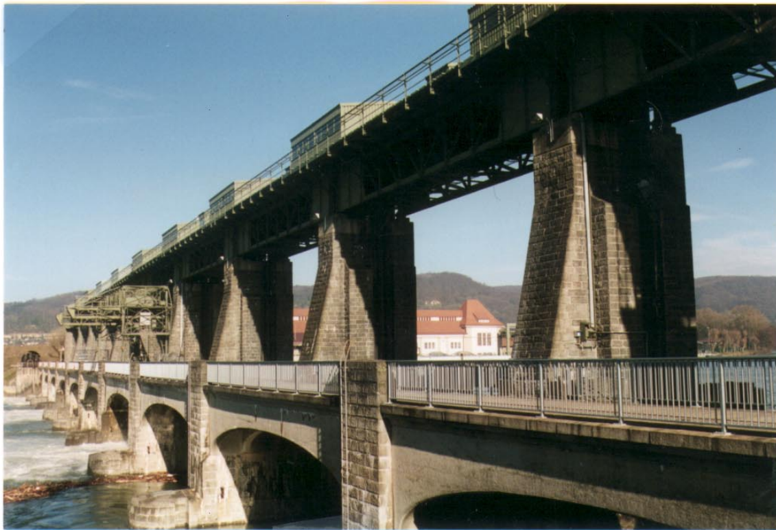
Fig. 1 Augst-Wyhlen Hydro-Power Station.
