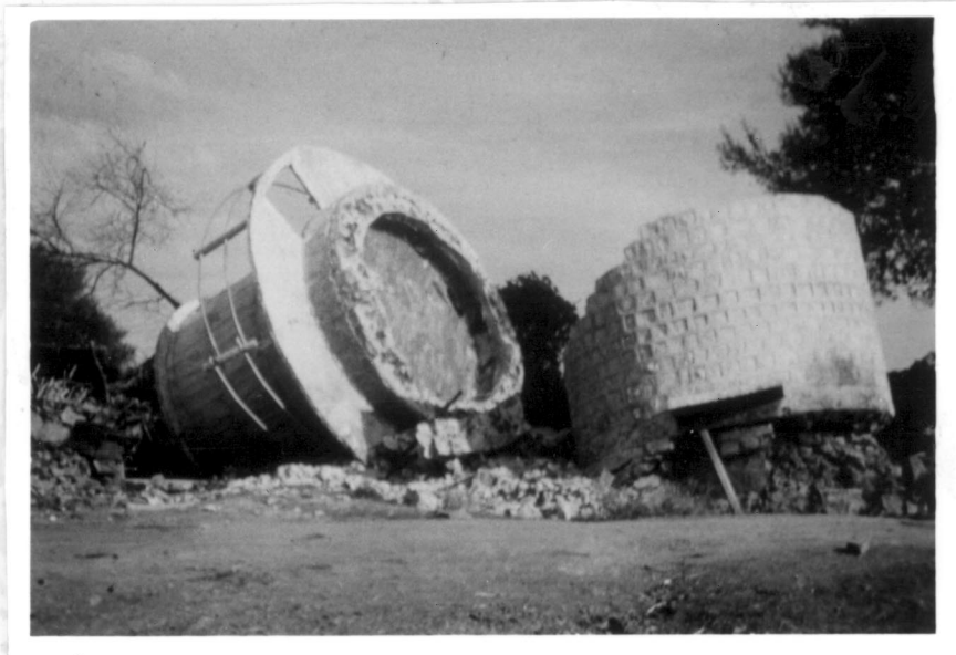
Photograph 10. Collapsed water tank at Chincholi (Rebe) 3 km from epicentre
