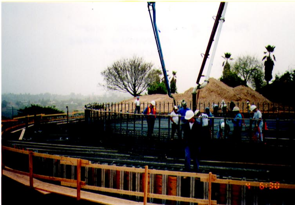
Figure 4 - Concrete Mat Foundation Under Construction
