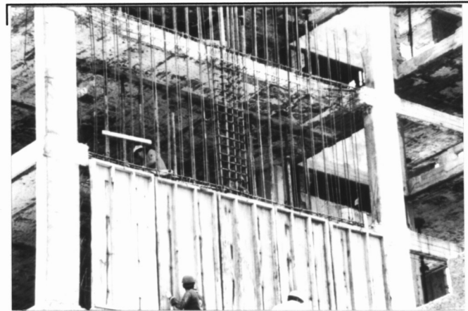
Figure 6. Reinforcement of new shear wall.
