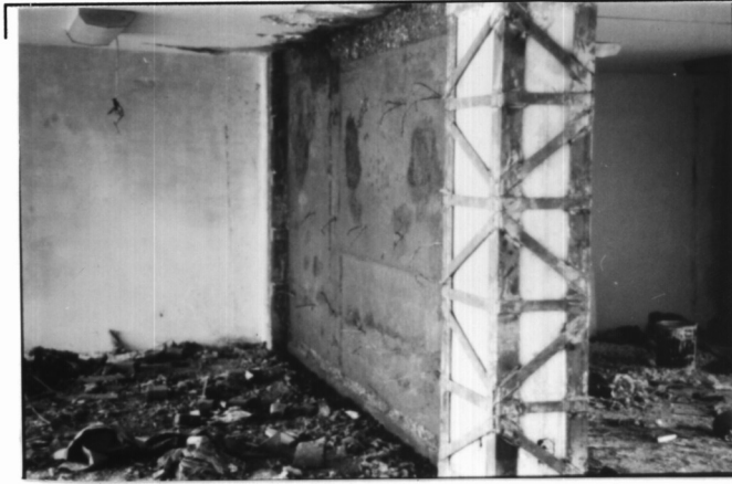
Figure 5. Jacketing of column with angles and straps.
