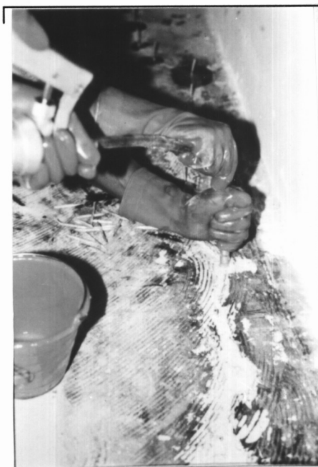
Figure 3. Crack injection of a damaged slab.
