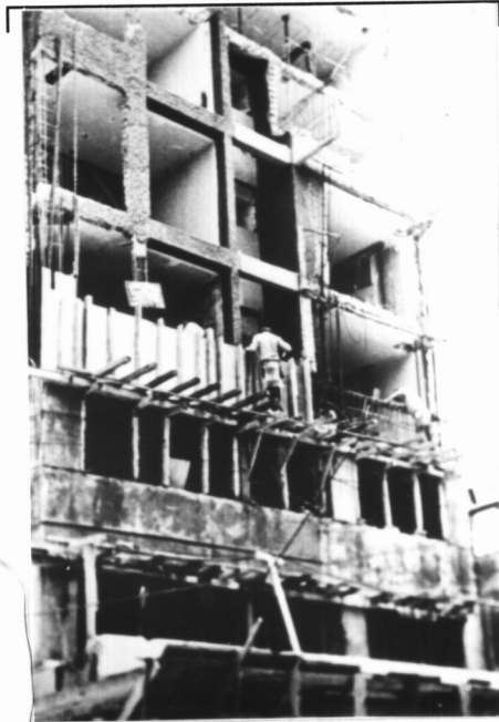
Figure 7. Addition of a reinforced concrete frame.
