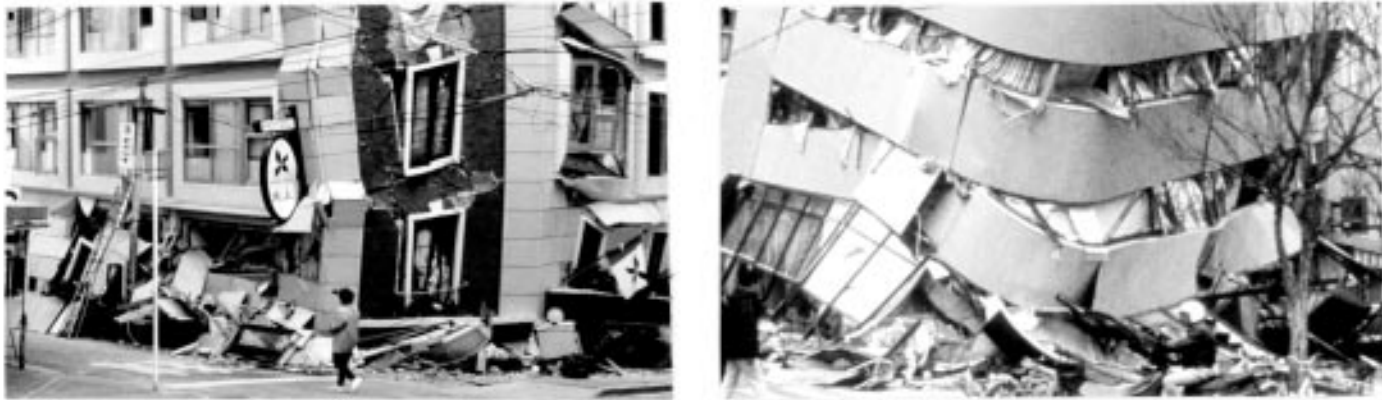
Fig.3 Soft first story failures: Kobe, Japan, 1995
