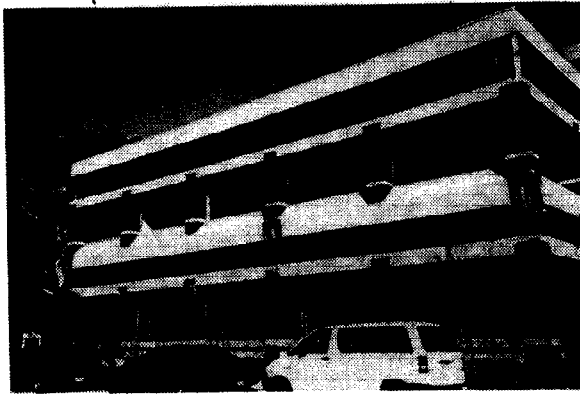
Fig. 1 Two Story Building
