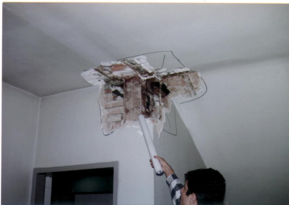
Fig. 3. Establishing Existing Members Used in Original Design
