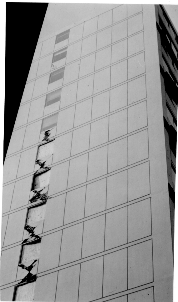
Fig. 1-Damage to the coupling beams of Champagne Towers
