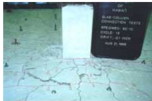
Figure 8: Punching shear failure, 1C.
