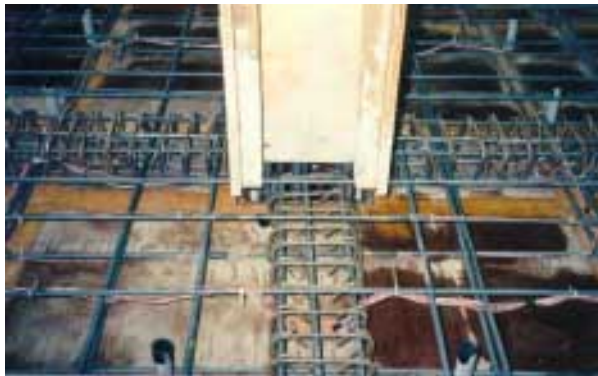
Figure 3: Closed hoop stirrups – Spec. 2CS
