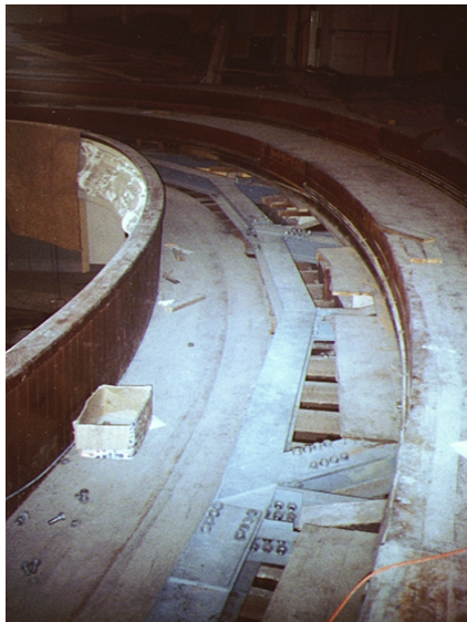
Figure 8: Circle Truss Inner Chord within Circle Bleachers
