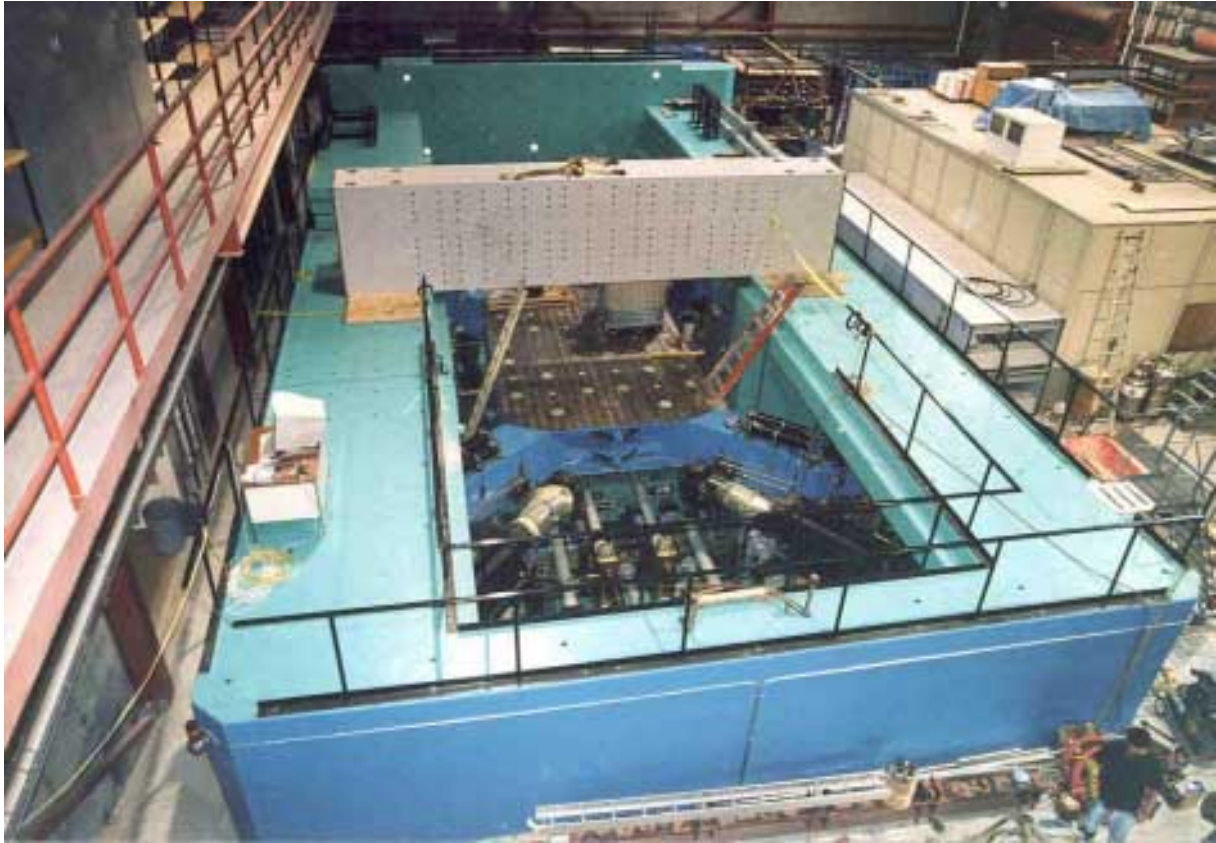
Figure 7. Completed Horizontal Reaction Frame, Platen and Hydraulic Distribution System
