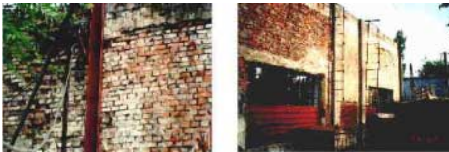
Fig. 7. Exterior images after strengthening
