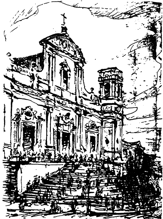
Fig. 02: The Cathedral of Reggio Calabria before the 1908 earthquake
