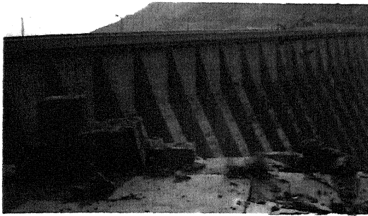
Fig. 3 Sefid-rud dam. Partial view of downstream.
