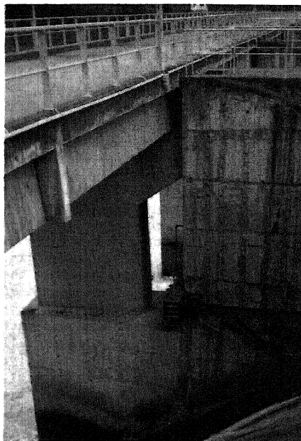
Fig. 8 Tarik dam. Details of the piers and the bridge deck.
