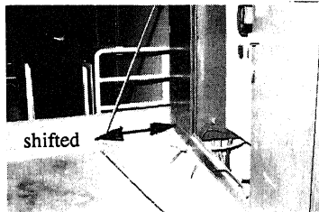
Fig. 3: Type-3 Pounding Damage Example.
