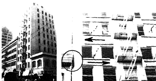
Fig. 1: Type-1 Pounding Damage Example.
