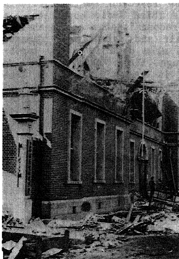
Figure 2. Damage of Mino-Owari earthquake, 1891 to unreinforced brick masonry building (Nagoya post office)
