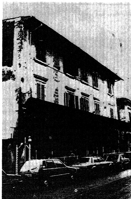
Fig. 1: Overall view of the building
