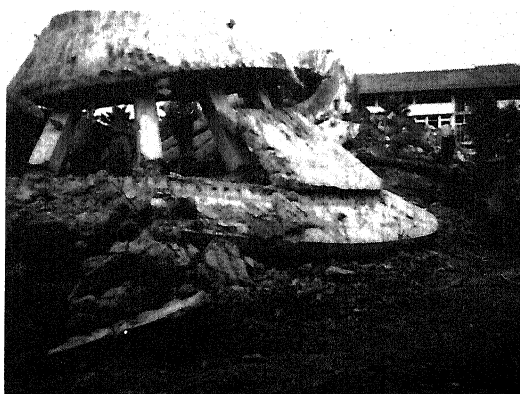
Figure 6. Total collapse of elevated water tank 1500 m 3 in Rasht
