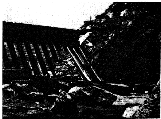
Figure 1. Buttress Sefidrud Dam built near fault. Experienced cracking at the interface of crown and tops also longitudinal crack has occurred.
