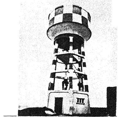
Figure 8 - General view of the elevated water tower in Lajes.
