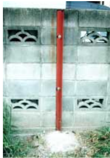
Figure 10: Existing wall strengthened with steel pillar
