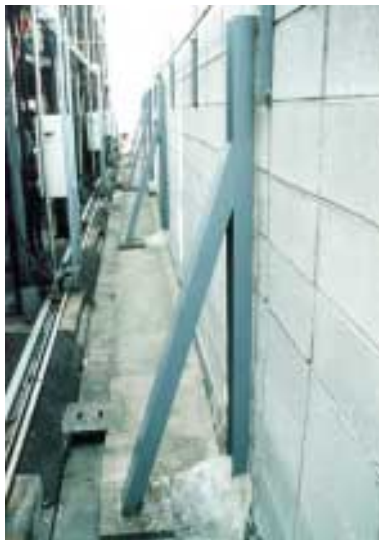
Figure 11: Existing wall strengthened with steel pillar and diagonal member
