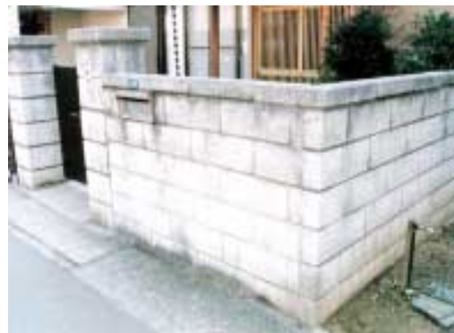
Figure 6: A wall having intersecting wall
