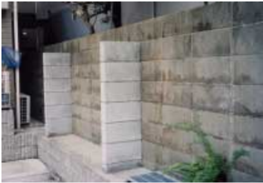
Figure 9: Existing wall strengthened with concrete block buttress wall
