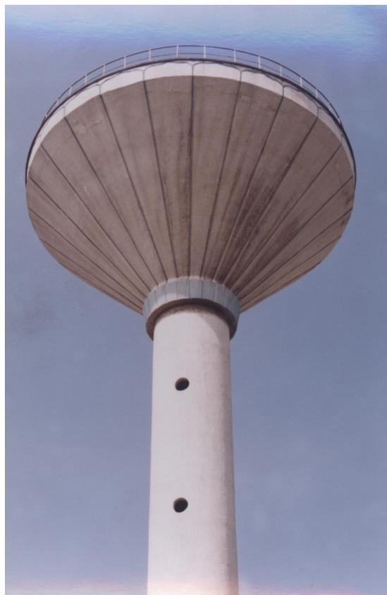
**Figure1: A Typical "Pure" Conical Tank**
