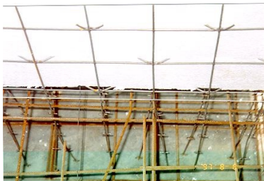
1. Wall and Foundation Anchorage
