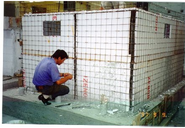
4.Specimen During Construction
