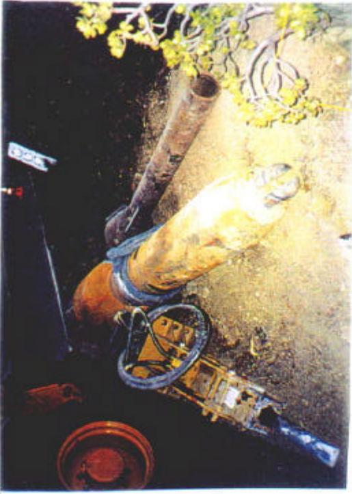
Figure 6-Pipe bursting tool assembly (pneumatic pipe bursting tool, expander cone and guiding sleeve) (L. Lund)
