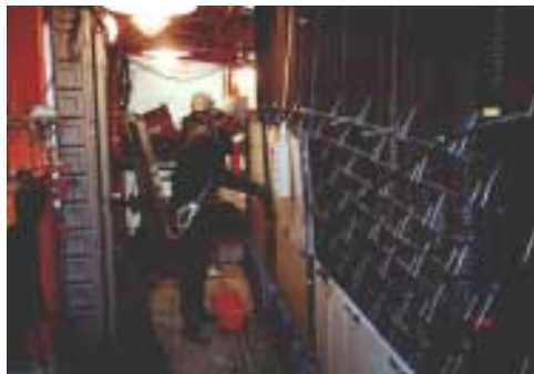
Figure 18: Installation of sheet-in-form
