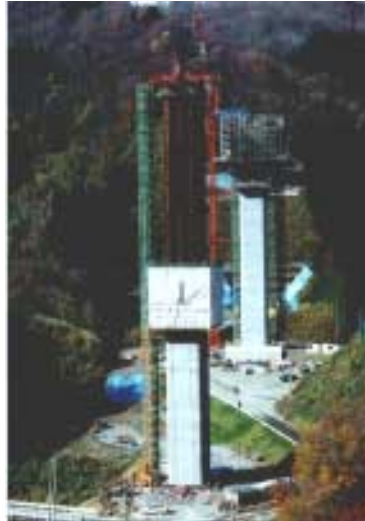
Figure 17: Hybrid-Slipform method construction
