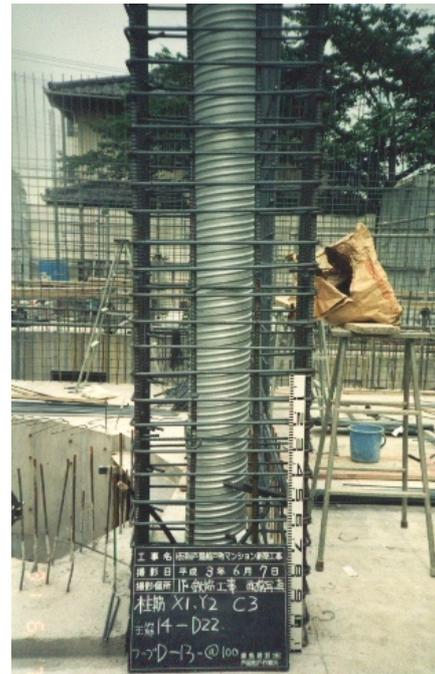
**Photo 1: actually constructed thin steel tube**
