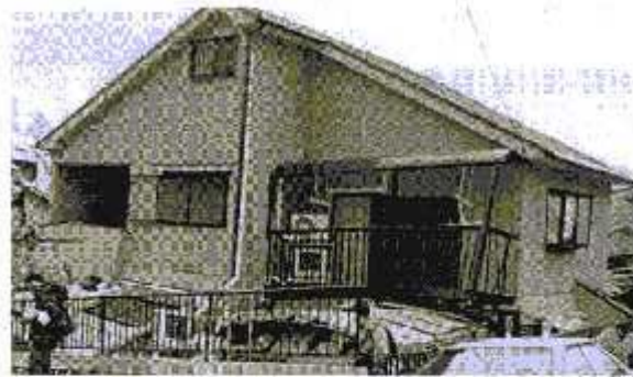
Photo.1 Collapsed 2 story house in Kobe
