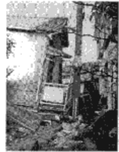
Photo.3 Seismic damage of S32-House in Kobe
