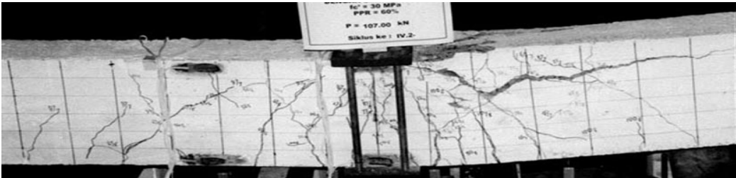
Figure 3. Crack Patterns of Original Specimens
