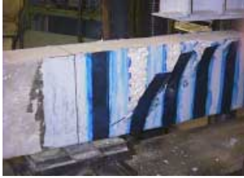
(a) Specimen A-SO3-2 (Debonding of CFRP over shear crack)
