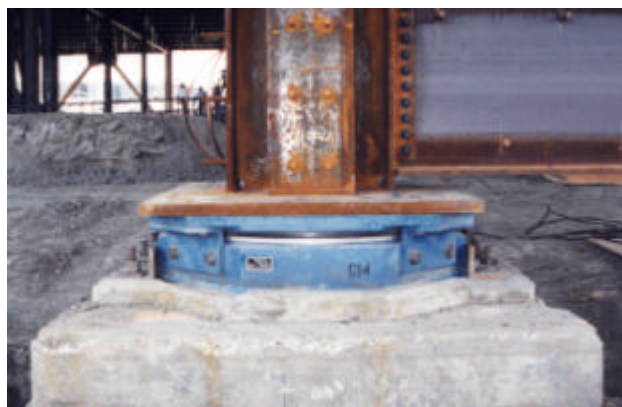
Fig. 6: San Francisco Airport Bearing Installation
