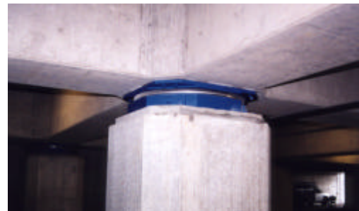
Fig. 16: Installed Bearing, Hayward City Hall
