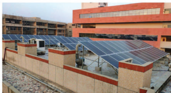
RENEWABLE ENERGY GENERATION THROUGH INSTALLATION OF 200KW SOLAR PANELS
