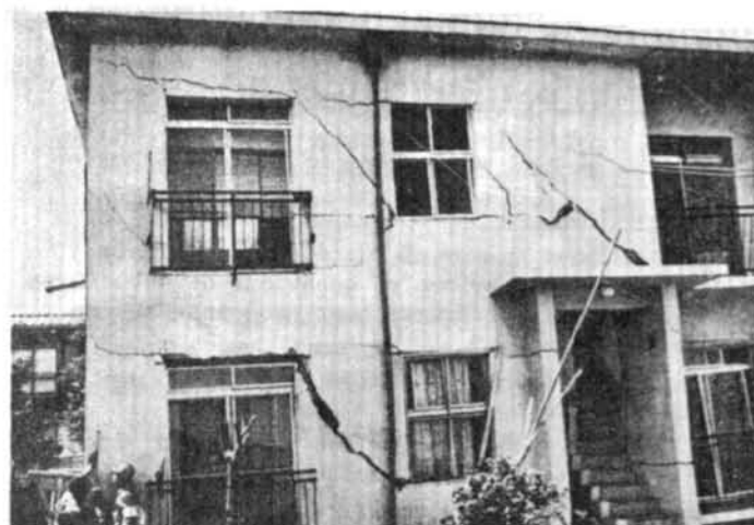
Plate 4-23. Cracks in this concrete block building were caused by differential settlement.
