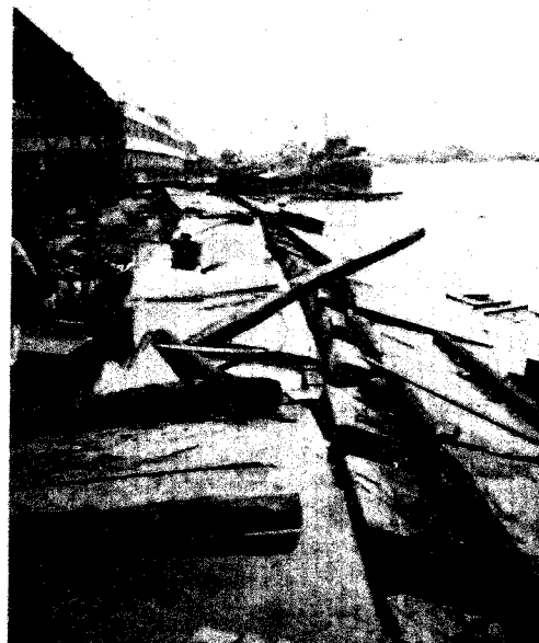
Plate 3-5. Damage to sheetpile quaywall reaching a depth of 4.0m.
