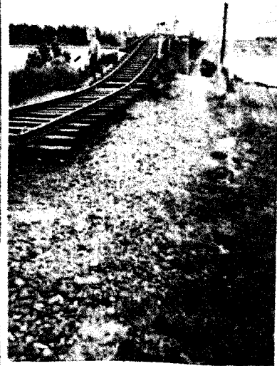
Plate 3-11. General subsidence of railroad embankment on old riverbed.
