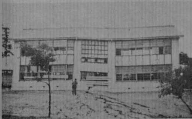
Plate 4-5. A wooden school building. The stairs in the center settled.
