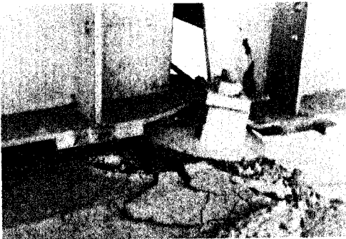
Plate 3-8. Damage to a support at Yachiyo Bridge. (A roller support on the left side)
