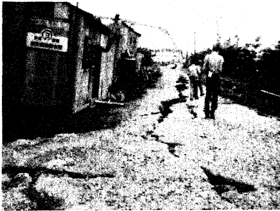
Plate 3-10. Longitudinal cracks in a levee.
