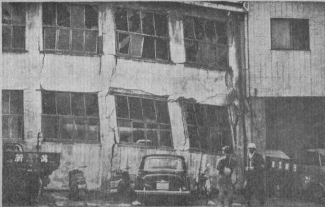
Plate 4-20. Failure near the junction between a two-story reinforced concrete building (on the left) and a three-story reinforced concrete addition.
