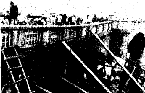
Plate 3-9. Deformed arch span at Bandai Bridge, viewed from the upstream side.
