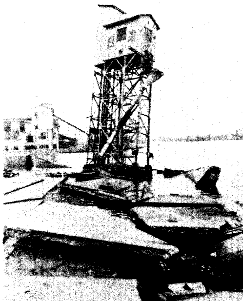
Plate 3-4. Damage at corner of South Landing Pier (concrete blocks) and South Pier (sheetpile).
