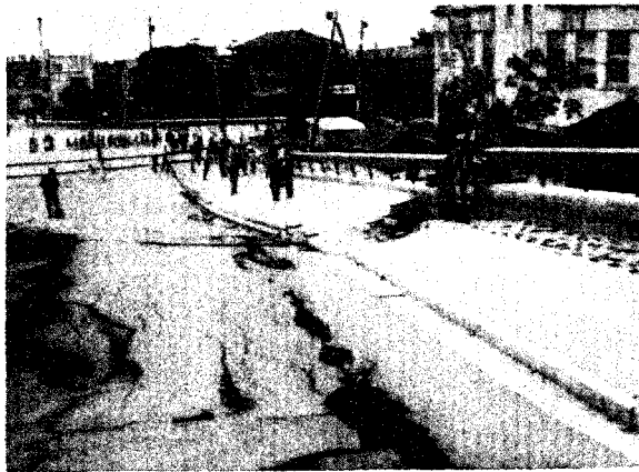
Plate 3-12. Subsidence of embankment at a bridge approach.
