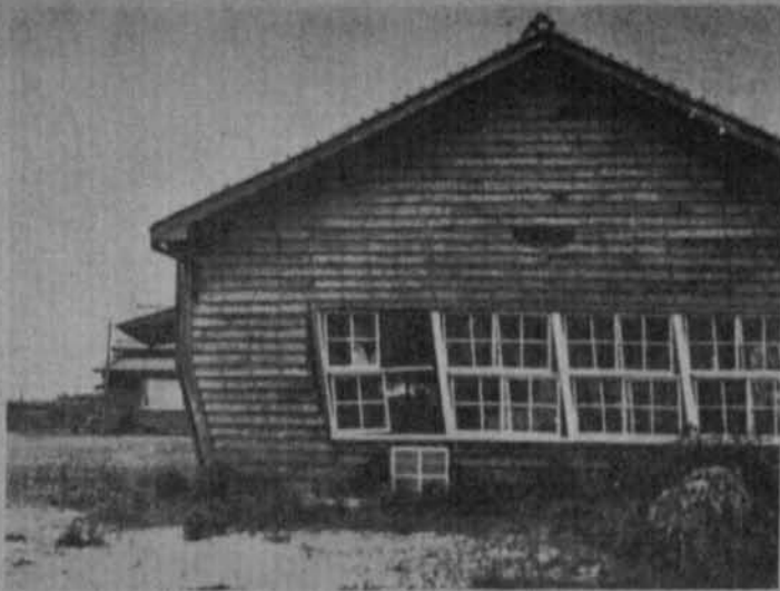
Plate 4-6. A warehouse. Columns were broken at braces.
