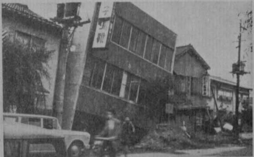
Plate 4-14. Large settlement (max. 2 m) and tilting (140/1000) of a building on 6-m timber piles designed to carry 6 t per pile.
