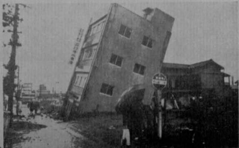
Plate 4-15. A large amount of tilting toward the heavier side of the building.
