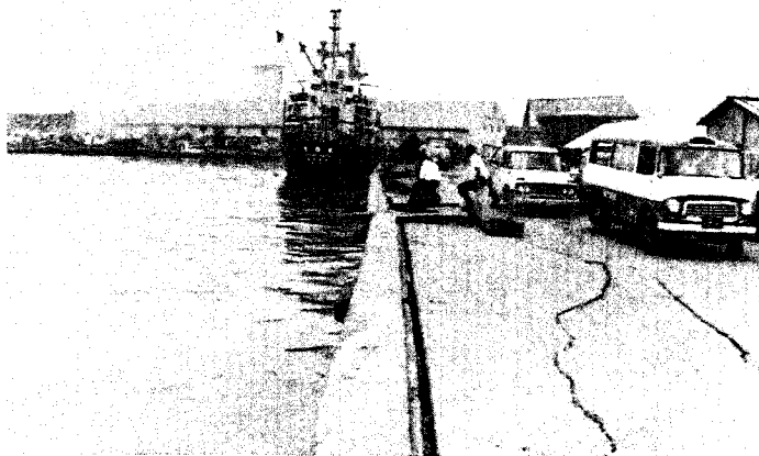
Plate 3-3. Damage to sheetpile quaywall at South Pier. Maximum settlement: 35cm; maximum translation: 2m.
