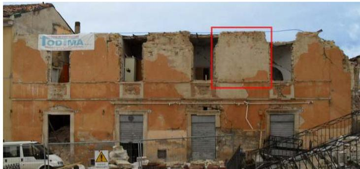
**Figure 1.1** View of the selected building and identification of masonry panel subjected to in-plane shear test.
