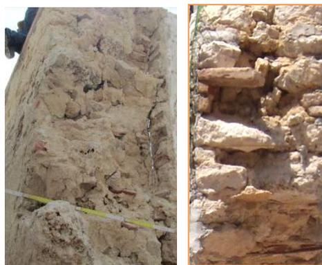
**Figure 1.2** Masonry cross-sections in the examined building.
