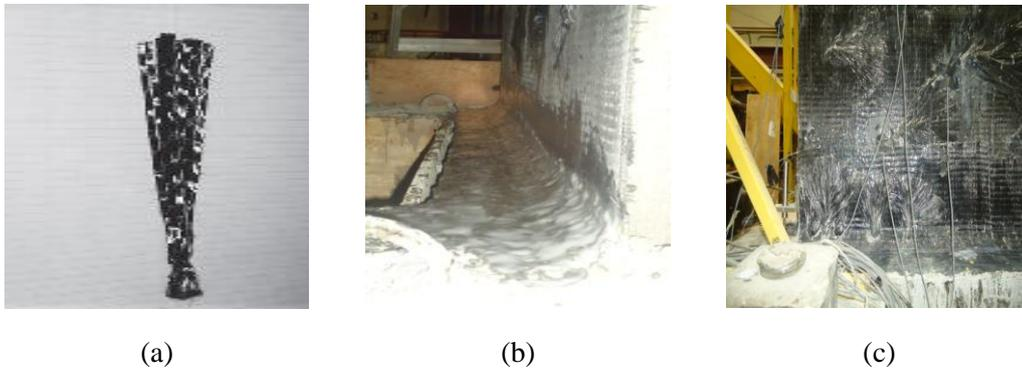
**Figure 3.** (a) FRP fan anchor (b) Rounding of wall-foundation joint prior to FRP application (c) FRP anchors in place.
