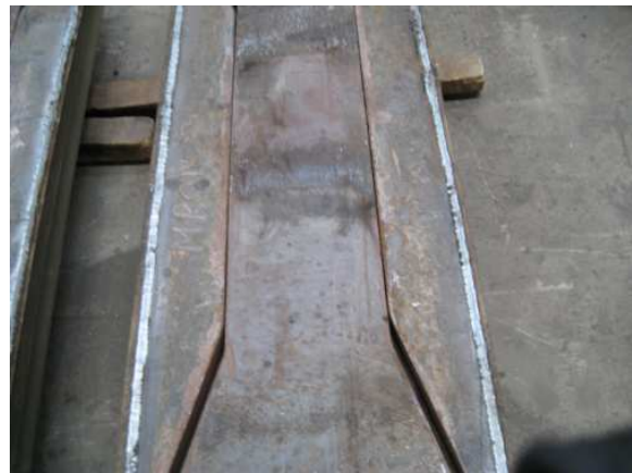
Figure 3.8. Open-up View of the Bottom End of the Left Energy Dissipation Segment of the All-Steel BRB After Testing
