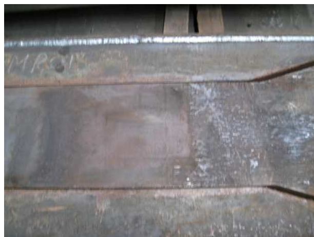
Figure 3.10. Open-up View of the Top End of the Right Energy Dissipation Segment After Testing
