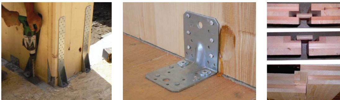
**Figure 1.** Hold-down, angle bracket and screwed-joints
