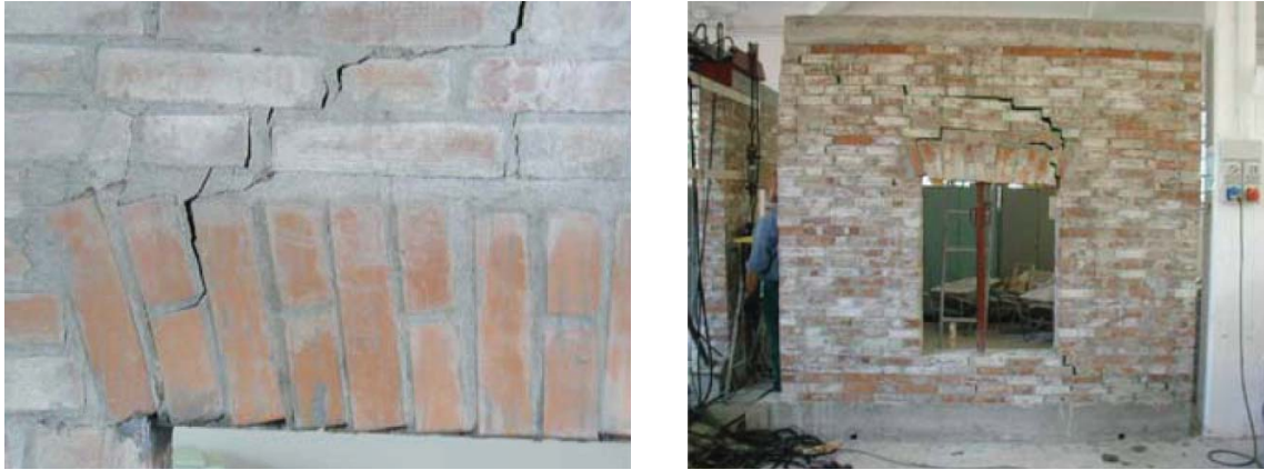
Figure 7. Crack pattern after test 1–3 and 3–5 (Foraboschi 2009)
